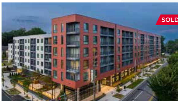
Gibson Reynoldstown Atlanta, Georgia 205 Units // Built 2022
