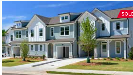
Brighton Woodstock Atlanta, Georgia 100 Units // Built 2022
