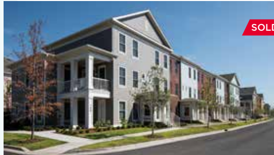
Veranda at Norton Commons Louisville, Kentucky 236 Units // Built 2015
