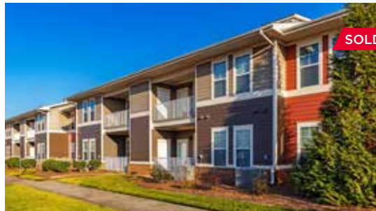
Lodge at Johns Road Huntsville, Alabama 83 Units // Built 2015
