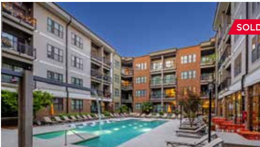
675 N. Highland Atlanta, Georgia 164 Units & 26K SF Retail // Built 2016
