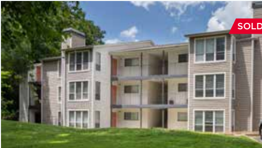
Equinox at Knight Fayetteville, Georgia 194 Units // Built 1988
