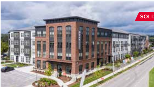
Accent Glassworks Nashville, Tennessee 282 Units // Built 2020
