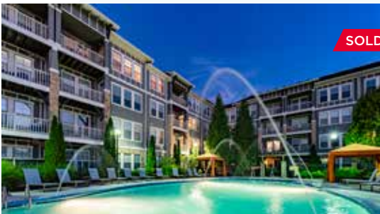
Regency at Johns Creek Walk Atlanta, Georgia 193 Units // Built 2012
