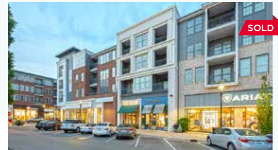
The Henry at Fritz Farm Lexington, Kentucky 306 Units // Built 2017
