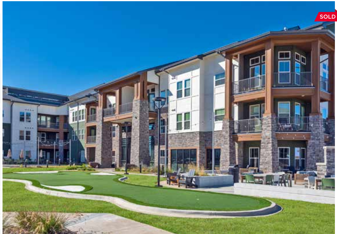
The Fitzroy Grove Rogers, Arkansas 250 Units // Built 2021
