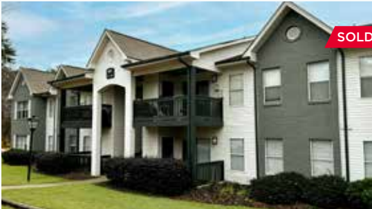
The Weathersby Charlotte, North Carolina 180 Units // Built 1996
