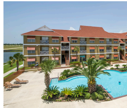
HARBORSIDE New Orleans, LA 168 units / Built 2004
