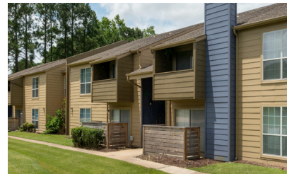
SOUTHERN OAKS Mobile, AL 224 units / Built 1975
