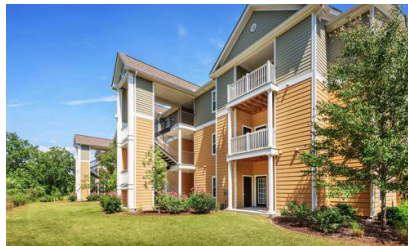
THE SUMMITS Graniteville, SC 120 units / Built 2012
