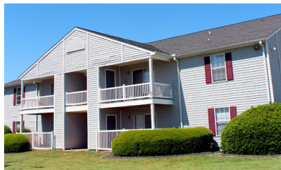
RIVER POINTE Robinsonville, MS 152 units / Built 1996
