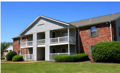
PECAN GROVE Walls, MS 152 units / Built 1996
