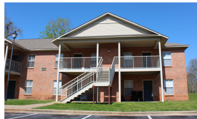
WINDING CREEK Tuscaloosa, AL 80 units / Built 1998
