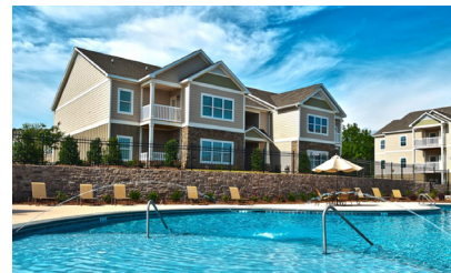
RIVERSTONE Macon, GA 220 units / Built 2012
