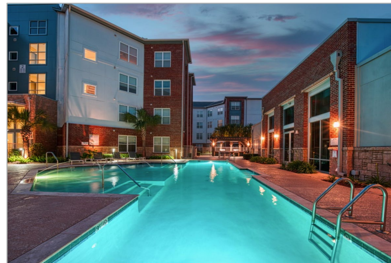
RIVER HOUSE Baton Rouge, LA | 266 Units | Built 2018 & 2022 (Phase I & II)
